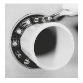
Manually tighten using a spanner or wrench only. Do not tighten any bolt more than 4 turns at a time. Tighten the bolts in a crisscross pattern or sequence until all bolts have been uniformly secured. Repeat this after a couple of hours to ensure long-term tightness of the bolts.
