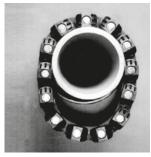
Ensure all bolt heads are facing the installer. Extra slack or sag is normal. Do not remove any links if extra slack exists. Note: On smaller diameter pipe, links may need to be stretched.
