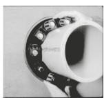
Slide the Micro Seal assembly into the annular space (ring-shaped cavity between the pipe and the wall). For larger size chains, start inserting the feedthrough at the 6 o'clock position and work both sides up toward the 12 o'clock position in the annular space.
