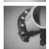
Loosen the pressure plate bolts just enough so the links can move freely. Connect both sections of the feedthrough around the pipe.
